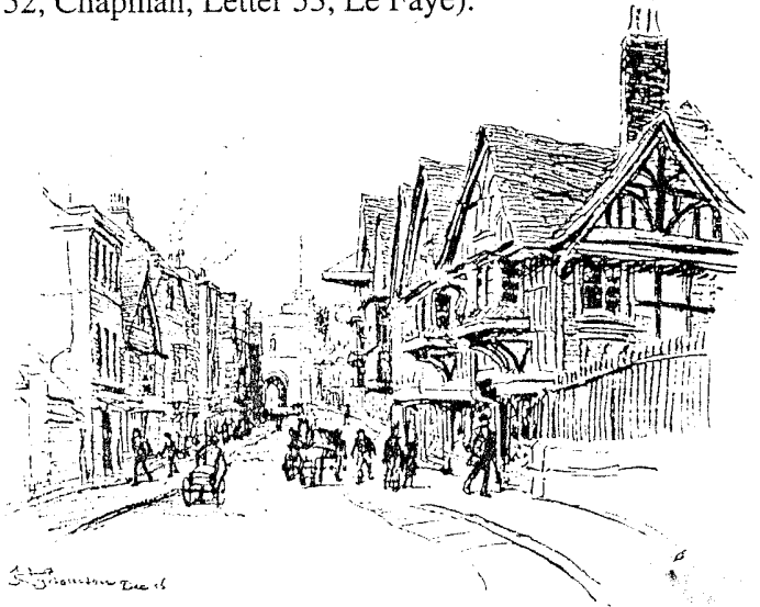
The West Gate from Within.
